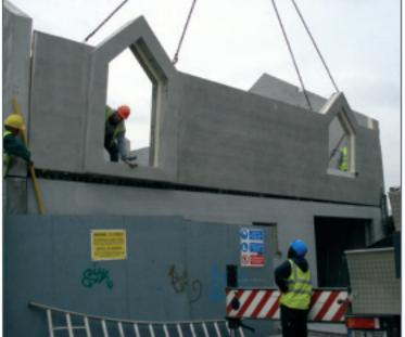
When the concrete has set the panels are lifted from the casting beds and placed in an upright position onto our unique Langendorf low level trailers for transportation to the site.
